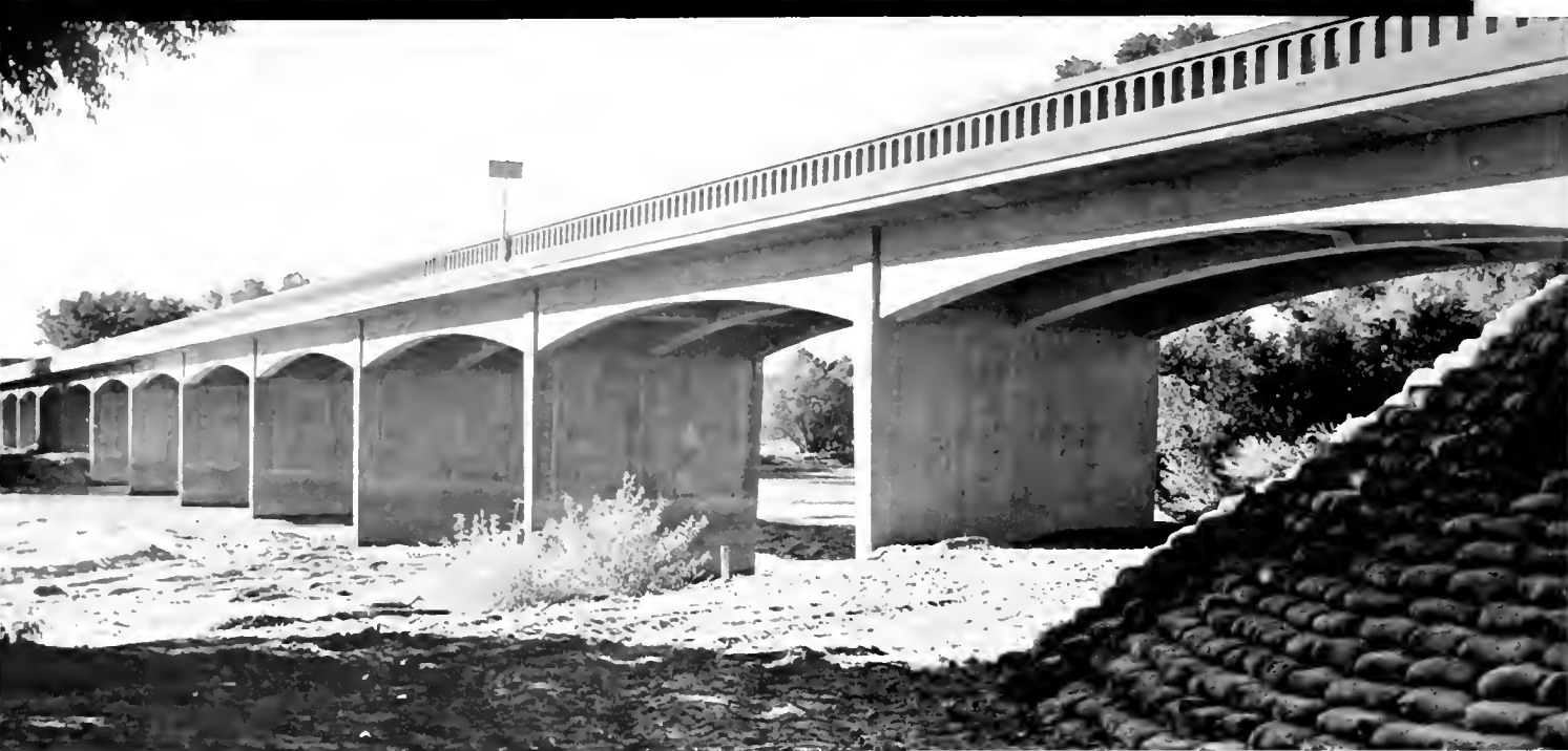
New Lanes Bridge across San Joaquin River on Fresno-Yosemite Highway is a 750-foot reinforced concrete structure
